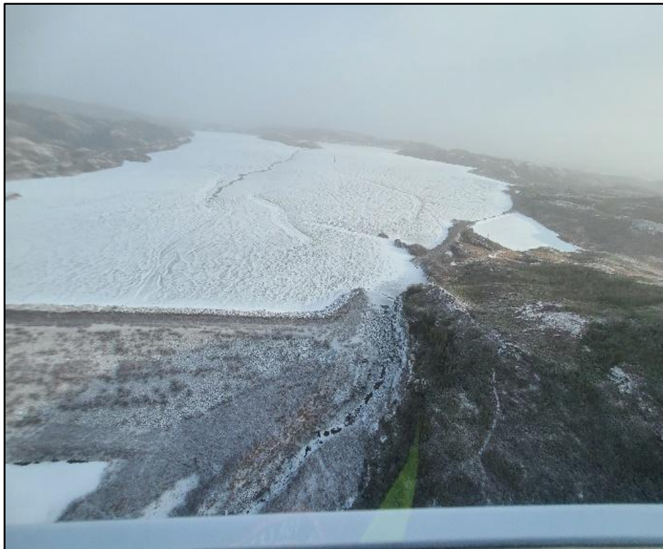
Figure 12-3: Main tailings dam showing overflow area to right
