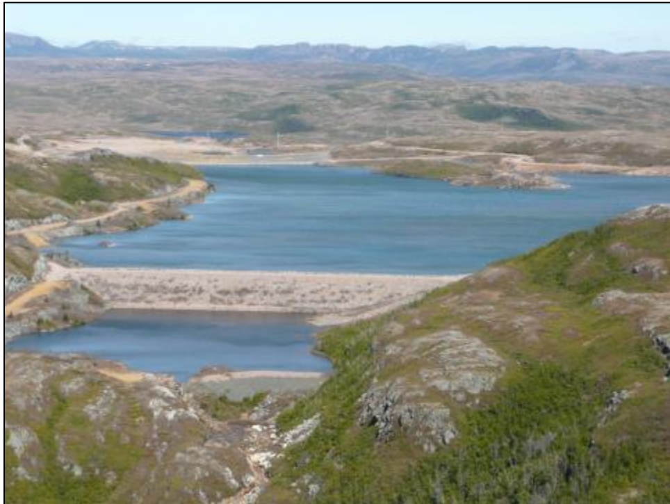
Figure 5-5: Main tailings pond facility at Hope Brook site
